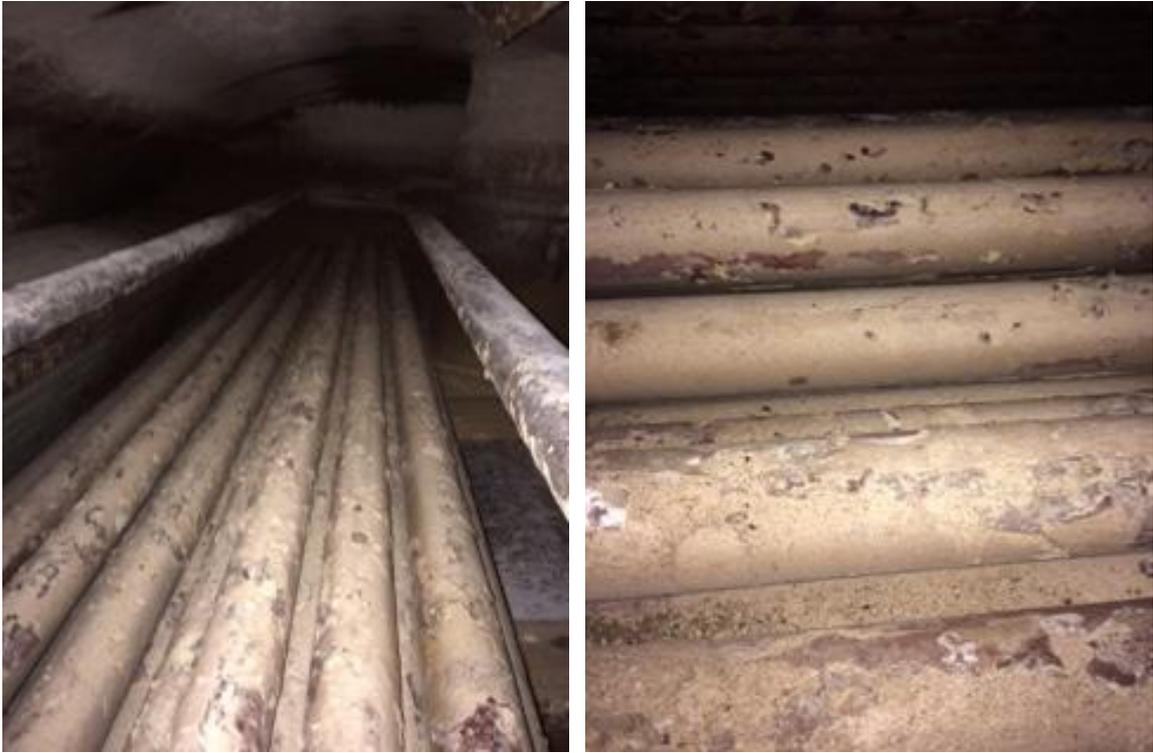
Picture 6 – Heat transfer surfaces after using ESC polymer technology
